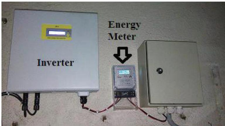
Figure 6. Inverter and energy meter
